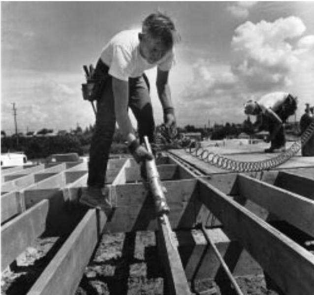
**Figure 9-6.** A pressurized extruder applies a single bead of elastomeric construction adhesive to floor joints for assembly of a plywood floor system.
